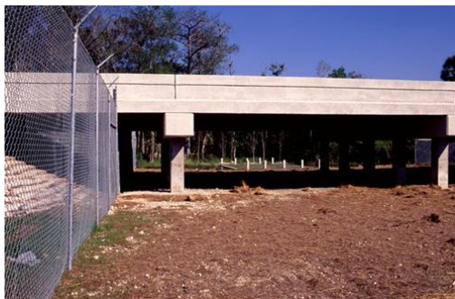
Figura 73. Paso inferior de fauna. Florida (copyright: Marcel Huijser). (Federal Highway Administration (FHWA), 2008).
