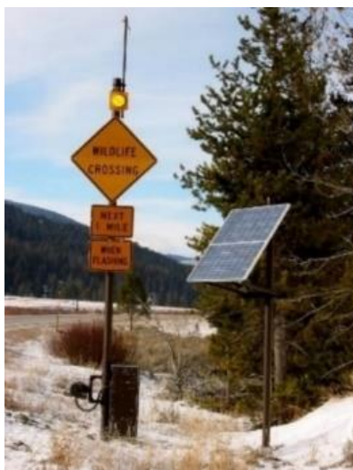
Figura 69. Sistema de detección de animales. Highway 191 in Yellowstone National Park, Montana. Photo by Marcel Huijser, WTI. (University, Huijser, Whisper, & Hardy, 2006).
